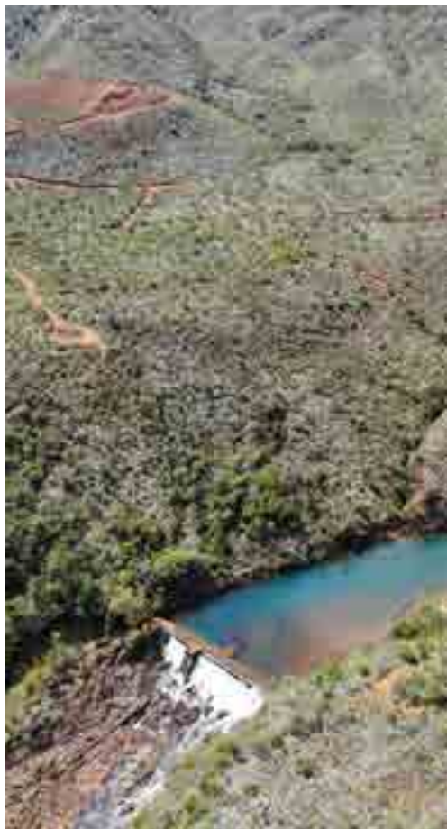
Barrage de Dumbéa – © D. Gonzalez
